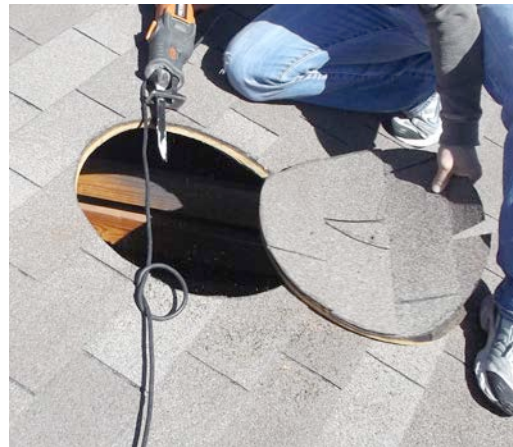
The hole cut out
