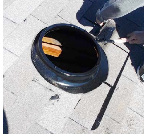
Sealing the flashing
