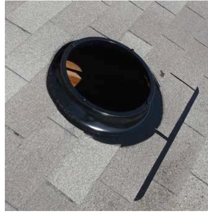
*Flashing after being slide in
