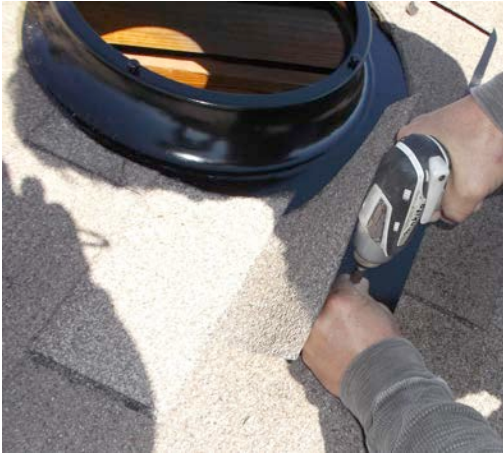
Securing the flashing
