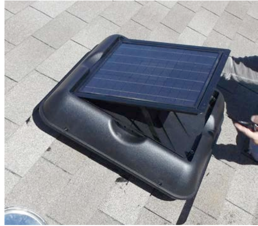
Raising the solar panel
