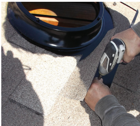
Secure the flashing
