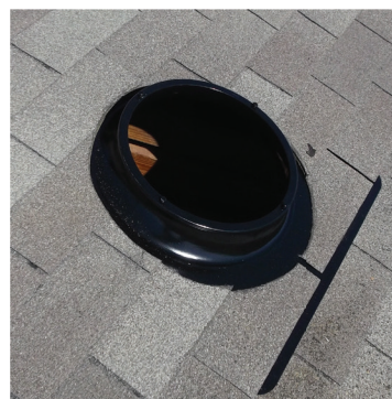
Flashing after sliding in
