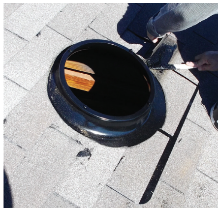
Sealing the flashing
