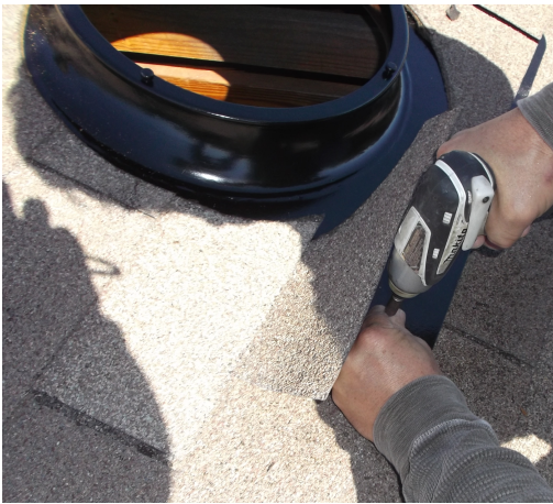
Securing the flashing
