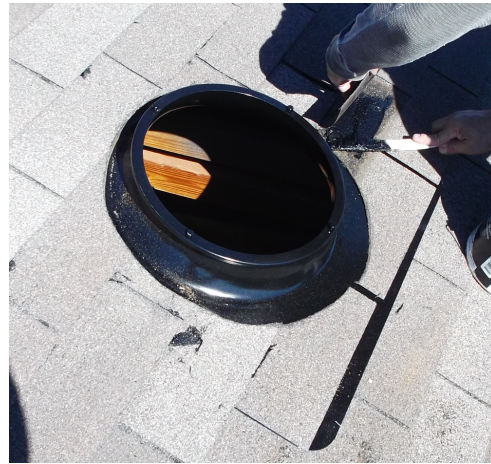
Sealing the flashing
